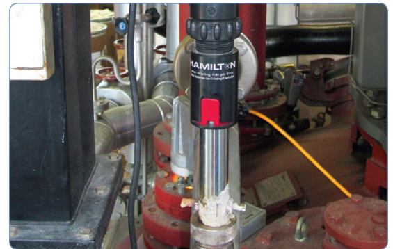
Figure 2: After more than 3 years of operation the Polilyte Plus H and RetractoFit are still in good shape and require only minimum maintenance.
