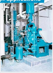
ABEL Compact Membrane Pumps are designed to handle difficult media: for all abrasive, corrosive, granular, pigmented or viscous products. Frequently, they are problem solvers under delicate operating conditions.
