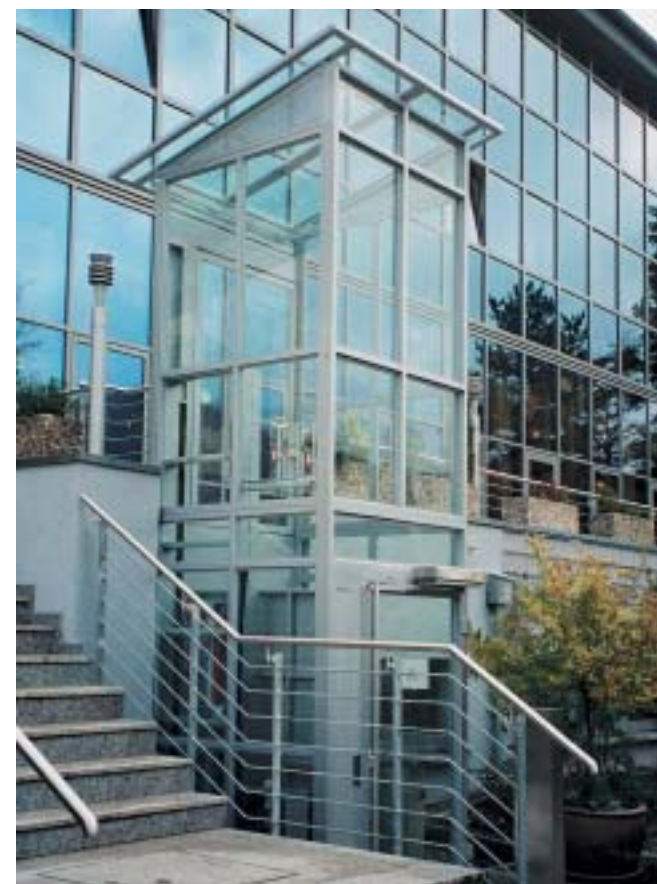
Column lift with glazed shaft.
