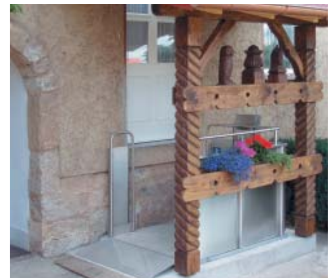
Corner layout with upper door on building.
