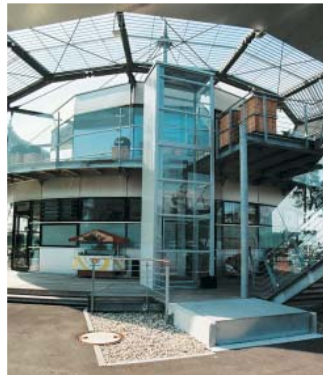
Access from terrace.
