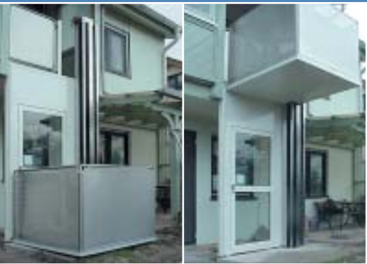
Installed with balcony access and an additional shaft wall.
