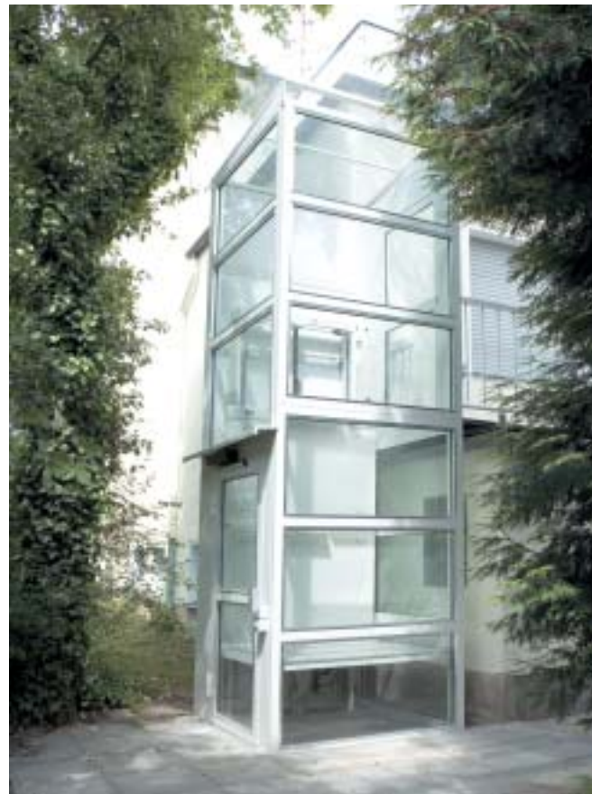
Lift with shaft panelled in safety glass and plastic.
