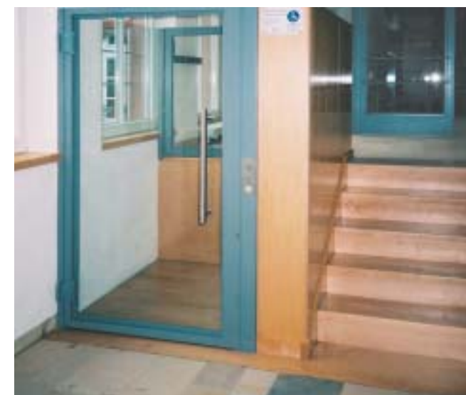
Lift with large glass door and wooden panelling.
