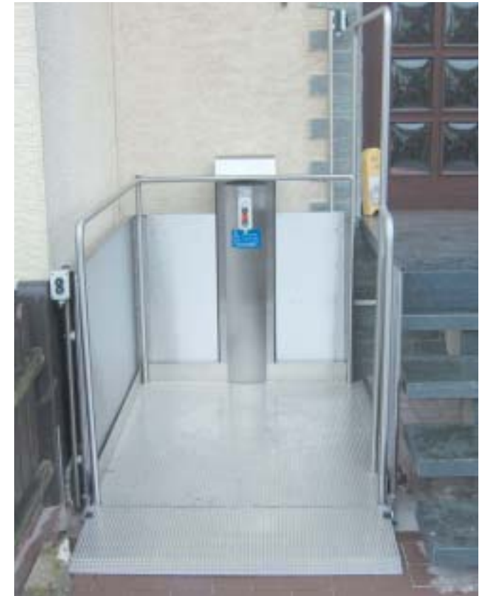
Corner layout with safety rails attached to lift.
