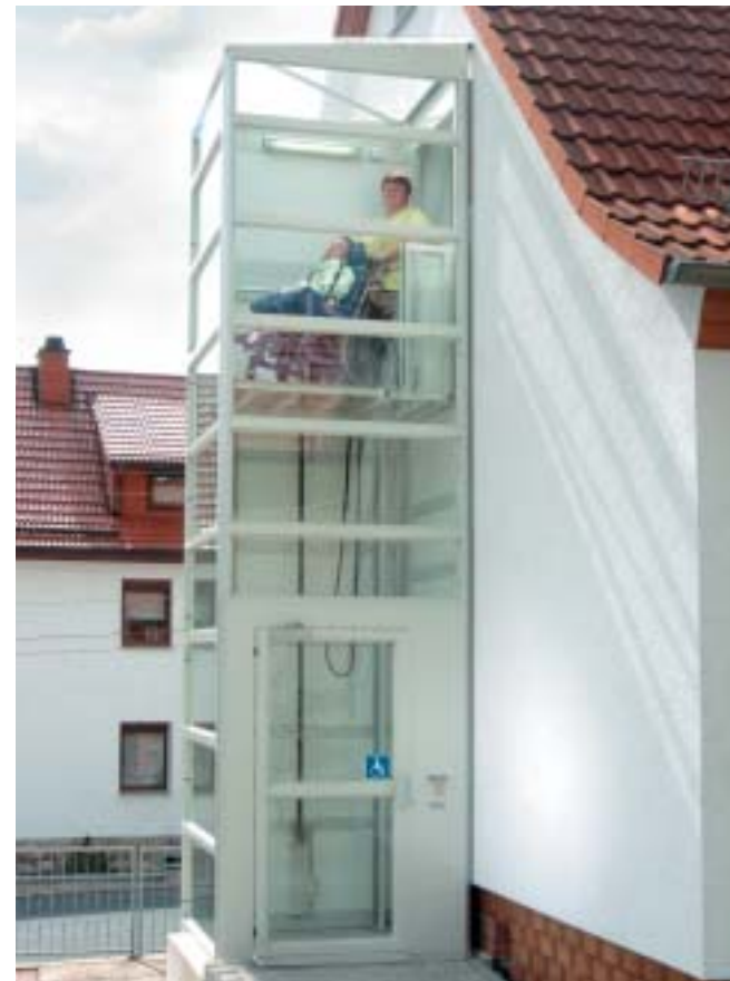
Outdoor lift under gable roof.
