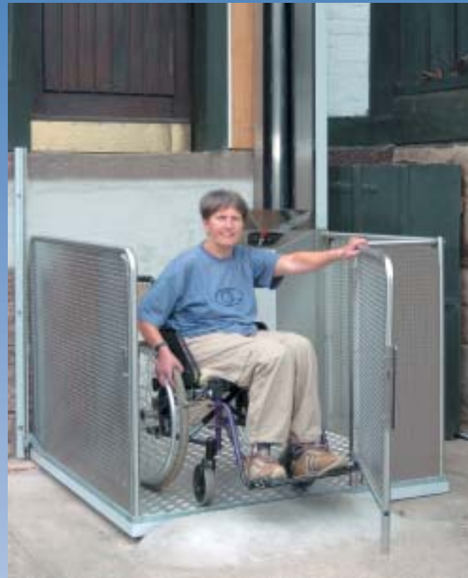
No-shaft lift with upper door on building.
